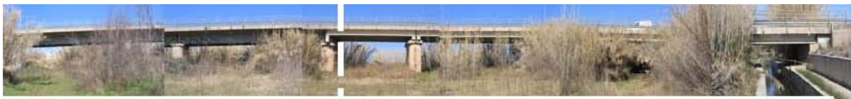
Figure 1. Photograph of the present bridge
