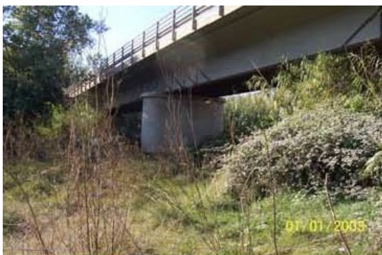
Figure 2. Extensions to the “pi” section and pre-stressed beams.
