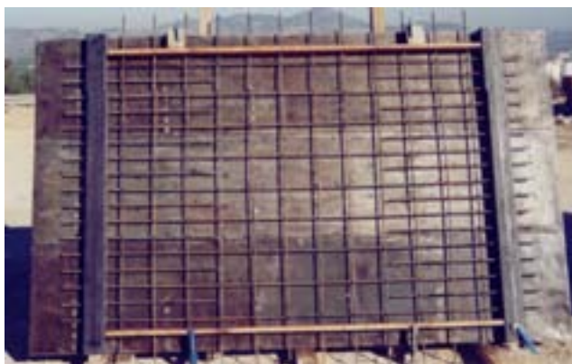
Figure 4. Shell specimen reinforcement
